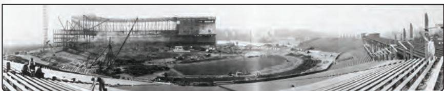
The original Yankee Stadium, shown during construction, was completed in only 284 working days.
